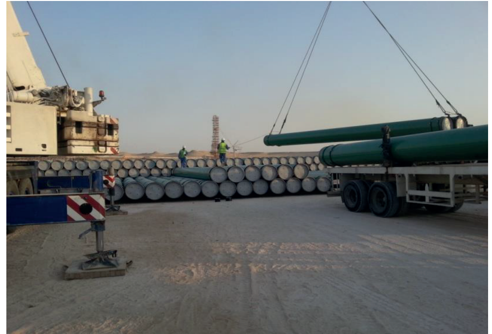
Being unloaded by crane using teflon coated pipe hooks
