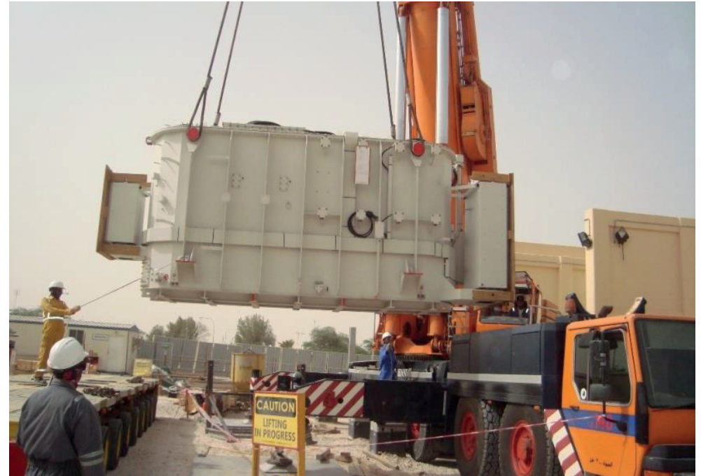
Lifting power transformer from trailer by mobile crane
