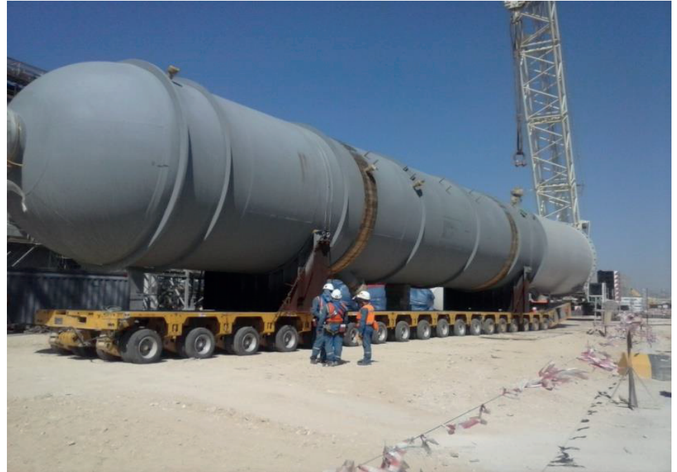
MSPM with HDS Reactor positioned near lifting area for installation at site
