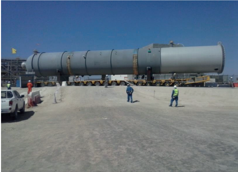
MSPM with HDS Reactor entering site
